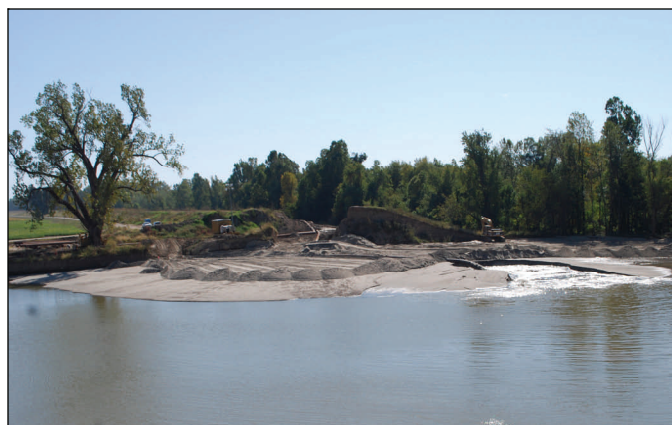
The dredge contractor pumps sand from the Mississippi River into the scour hole at the center crevasse Sunday.
