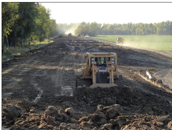
A Vicksburg-based crew repairs a 300-foot-long washout near the lower crevasse Sunday.
